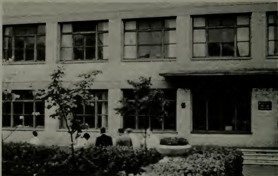
The workshop building at Kaschenko Hospital.
